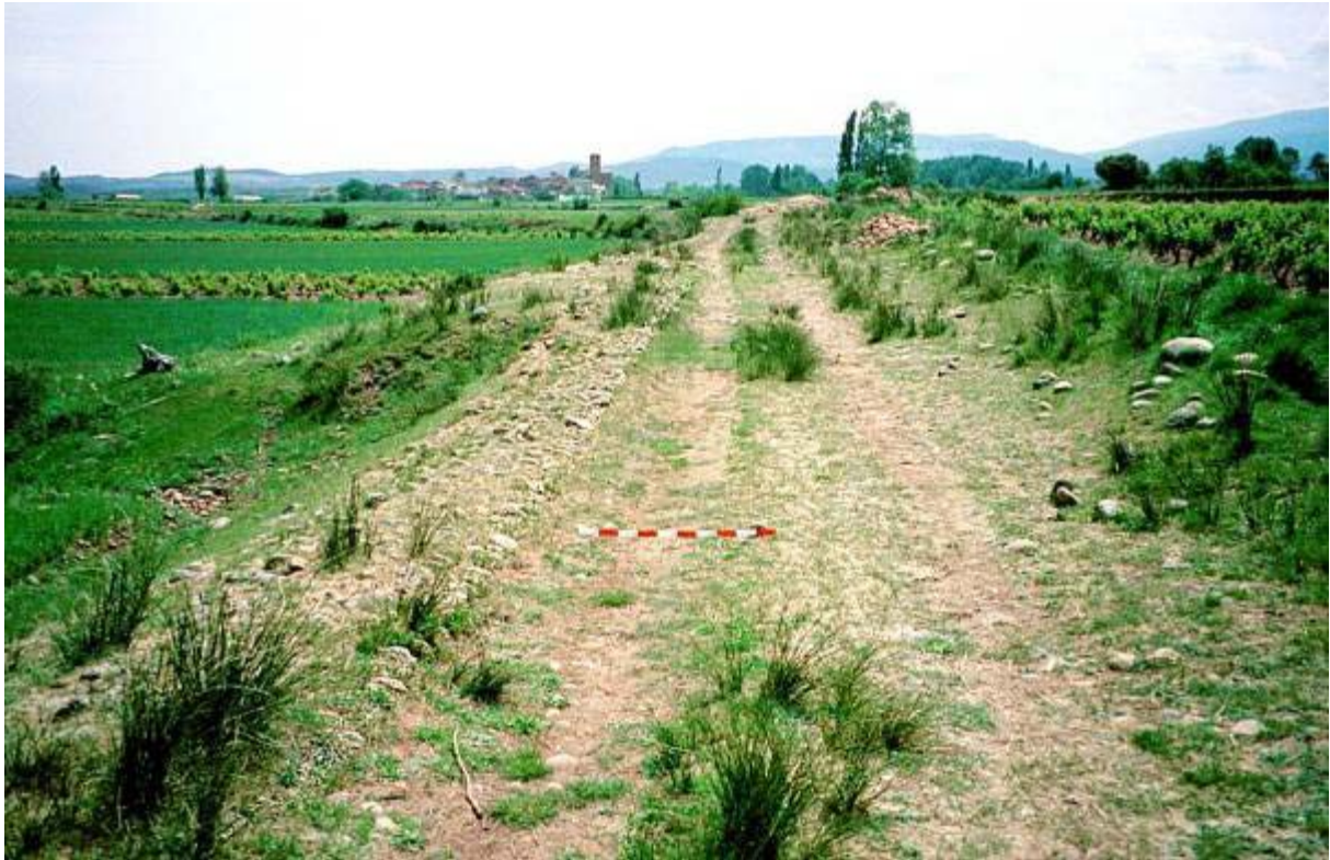
Perfectly preserved embankment with remains of upper kerb on the road from Italia to Hispania in Tricio. In the background, Alesón.
