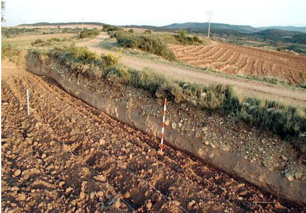
Detail of the thickness of the road surface in a side-section caused by the terracing of adjacent property. Roman road from Italia to Hispania between the hill of San Antón and Alesón.y Alesón.
