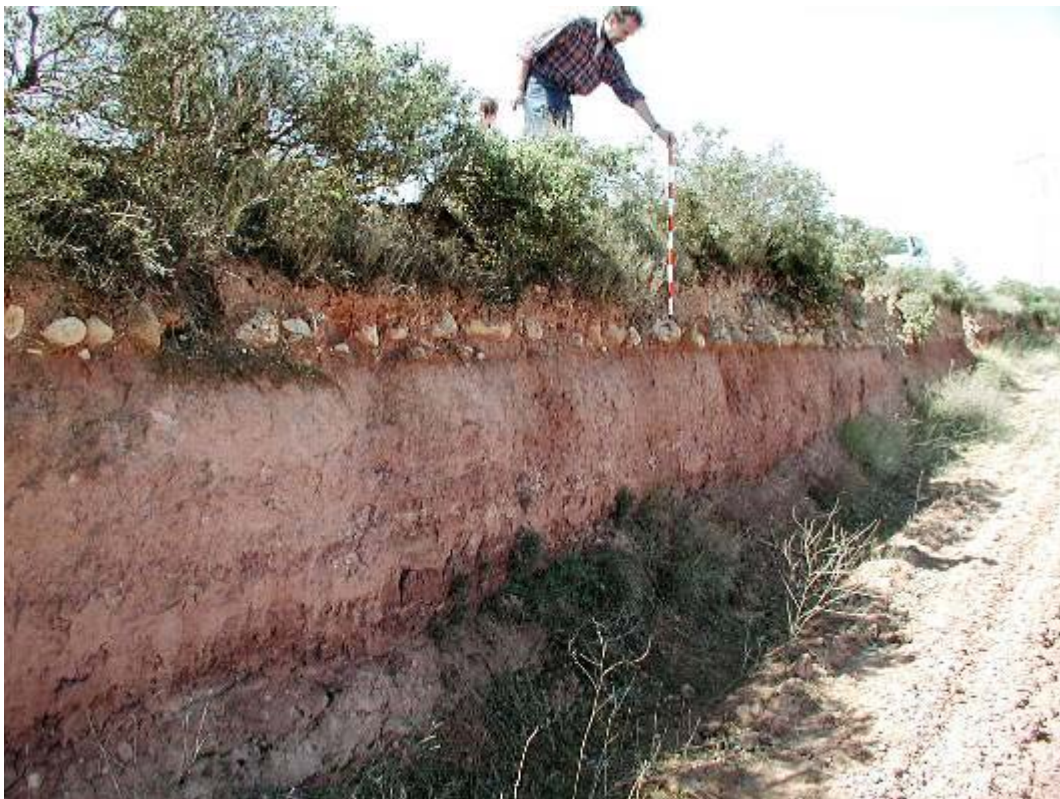
Foundation of round stones in a side-section caused by the terracing of adjacent property. Road from Italia to Hispania between the hill of San Antón and Alesón.
