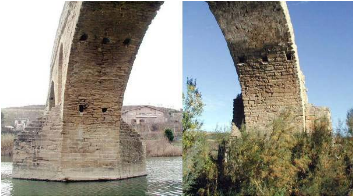
Detail of the bridge at Puente de la Reina on the left and that at Mantible. Note the size and irregularity of the bond, the width and proportions of the vaulting, the positions of the scaffolding slots, etc.
